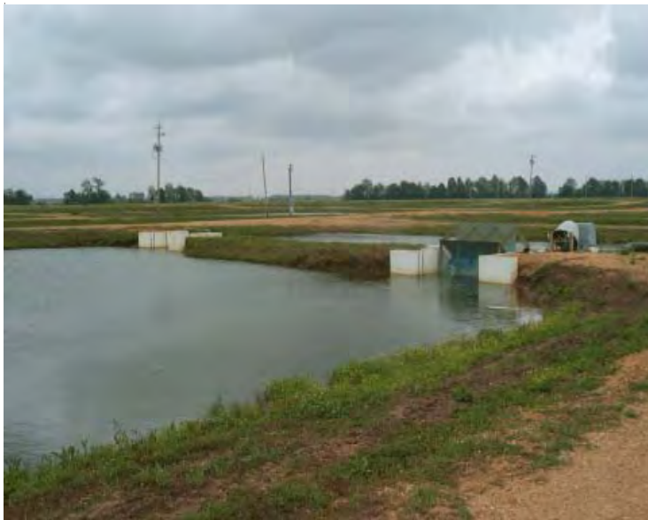
Figure 9. The split-pond system at Stoneville, Mississippi. An existing 0.32-ha earthen pond was split into a waste-treatment basin (foreground) and a fish-holding section (barely visible over the dividing levee). The two basins are hydrologically connected by a low-speed paddlewheel (at the right) and a return-flow sluiceway (at the left).
